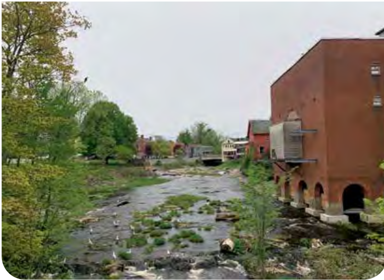
Exeter Great Dam in Exeter, New Hampshire before the dam's removal (2002) and after its removal in 2016. Credit: NOAA.
